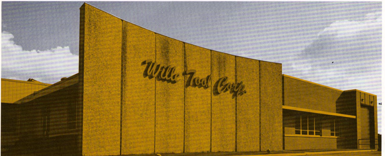
Wille Tool Corp. modern plant in Skokie, Illinois. New stamping area is at right.
